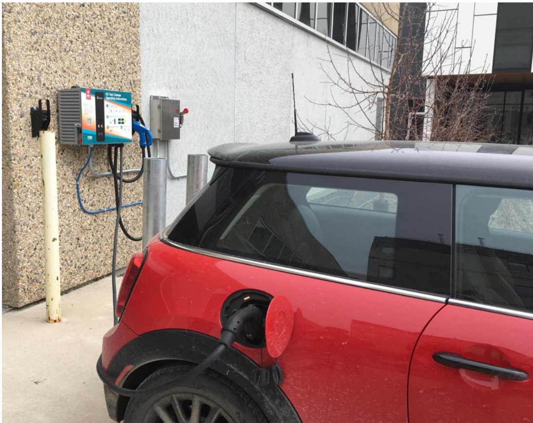
Figure 1. Exterior vehicle plug-points for B2U DCFC system at RRC Polytech showing an electric vehicle connected and charging. (R. Parsons 2022).
