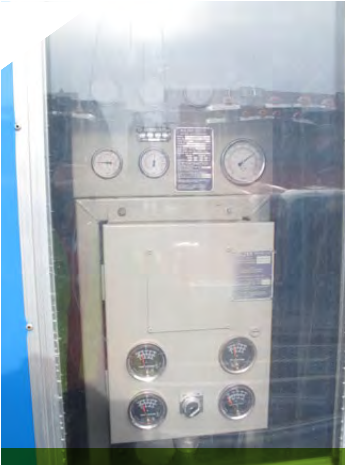
Figure 15 - View of Station Gauges
