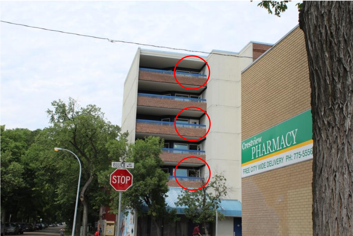
FIG 3: BUILDING #2 Location of blower doors in the balconies
