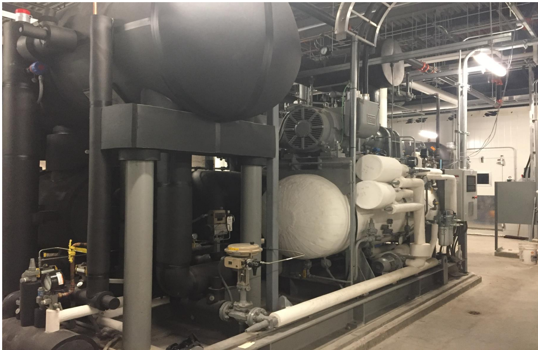
Main Low Temperature Chiller
